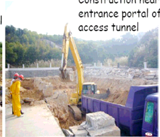
Ready to build construction tunnel
