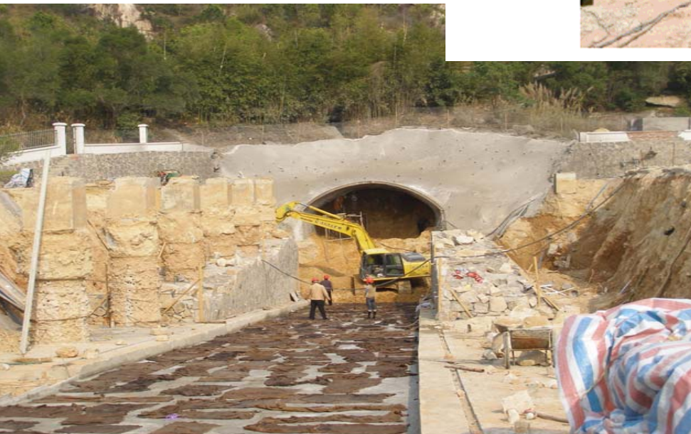
图片1： 进入隧道施工现场 February 2008, At the main entrance tunnel
