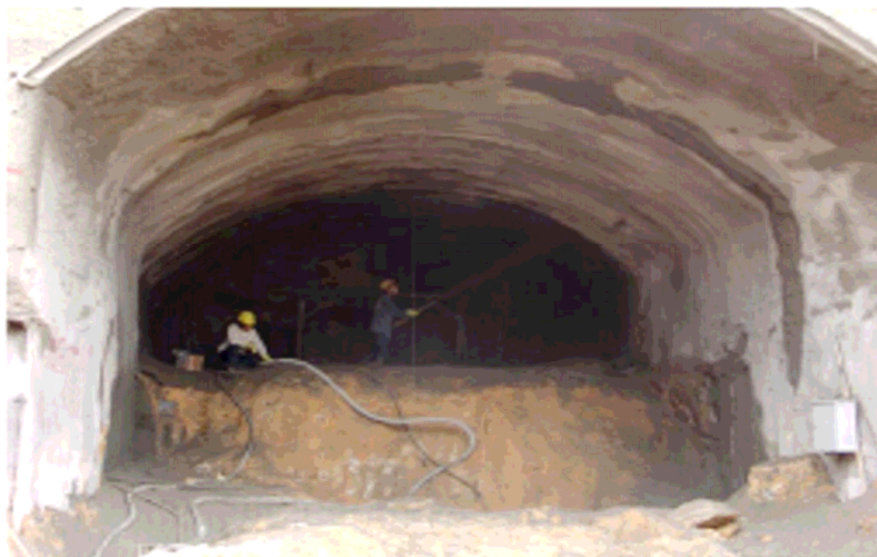
Daya Bay Main Access Tunnel
