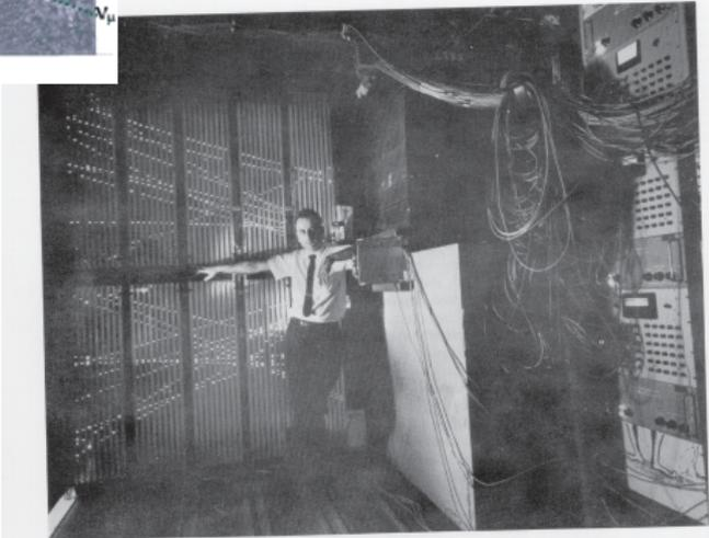
Mel Schwartz standing in front of the 10-tonne spark chamber used in the 'two-neutrino experiment'. Each of the ten modules contains 1 tonne of aluminium in the form of nine plates which are 2.5 centimetres thick and separated by a gas-filled gap of 1 centimetre. High voltage across the plates causes the gas to spark along the tracks of charged particles, which, in this time-lapse picture, are cosmic rays. (Brookhaven National Laboratory.)
